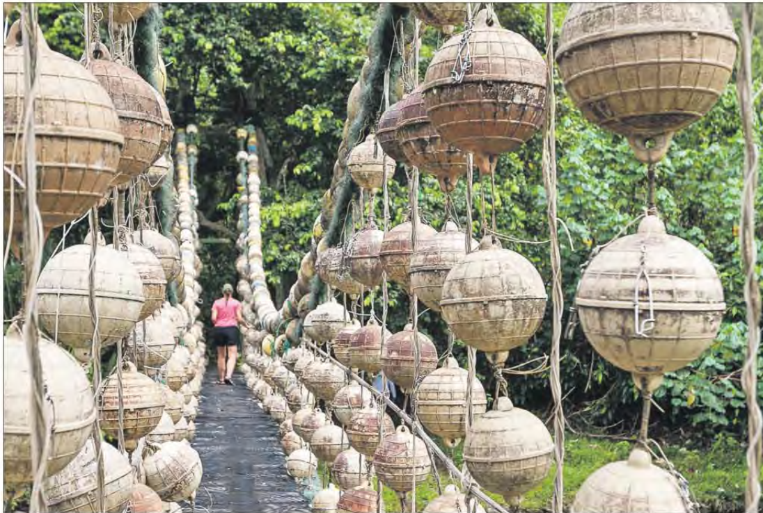
Cocos Island National Park rangers constructed this bridge entirely out of fishing line, buoys and other items confiscated from fishermen illegally working in the rich waters around the island nearly 350 miles off the Pacific coast of Costa Rica. ERIC MOHL • Special to the Star Tribune
